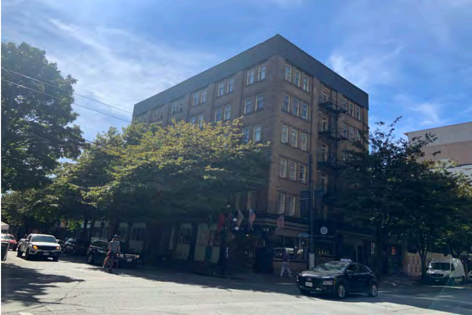
Subject Property looking southwest
