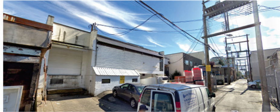
2- STREET VIEW: LOOKING NORTH-EAST
