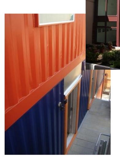
Texture was created by marrying the articulated Corten steel corrugated panels with opaque glazing panels and accented dashes of rich, clear-cedar horizontal siding and soffit.
