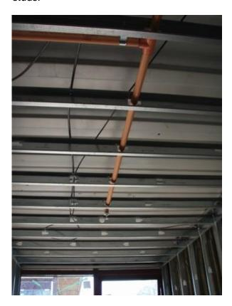
Although wood studs would have been more cost economical the proximity to adjacent and subsequent code provisions dictated a need for certain exterior walls to be constructed of noncombustible materials
