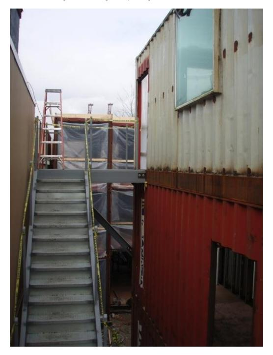
Modifying the container also required a significant amount of engineering to meet seismic / wind loads for code, design coordination and fabrication such as steel cutting and welding.
