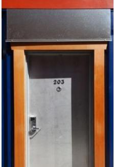
Doors are standard insulated metal installed and weatherproofed with appropriate caulking and custom designed metal flashings.
