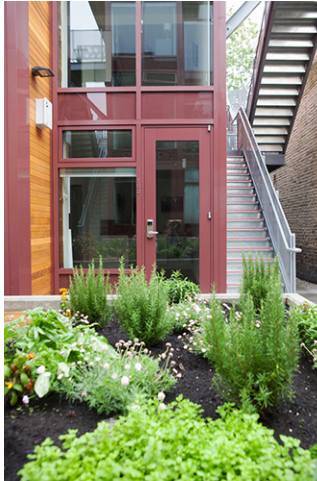
Image 2: View of Oneesan Container Housing from the site's courtyard (Source: Atira Women's Resource Society)
